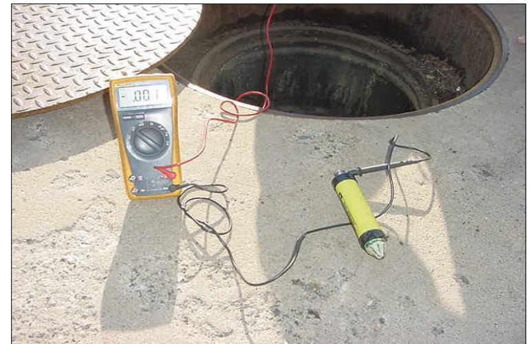
Voltmeter and reference cell used to perform cathodic protection tests.
