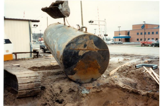
Tank removals were common in North Dakota prior to 1998.
