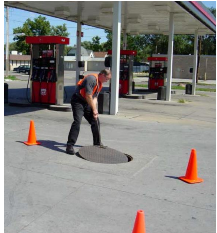
Opening a sump for visual inspection
