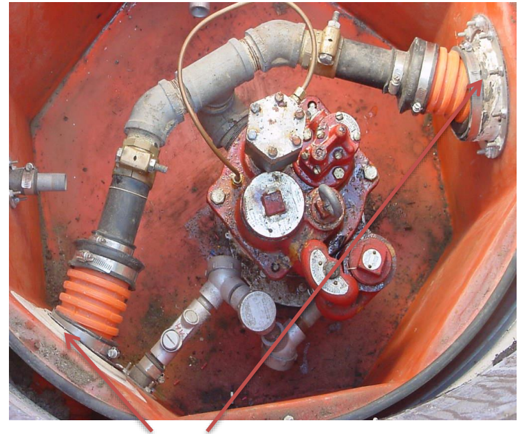
Sump penetration seals in good condition
