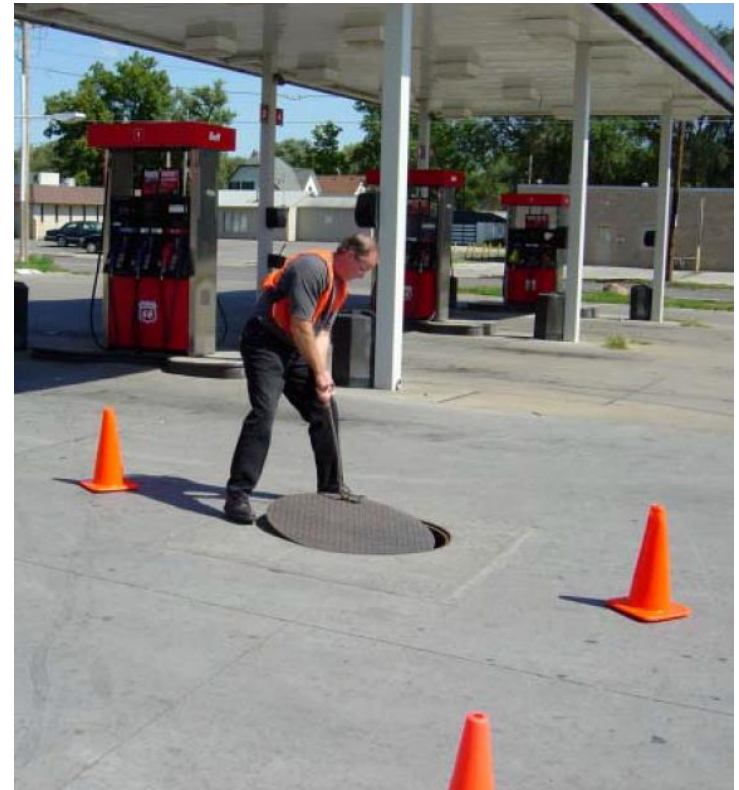
Opening a sump for visual inspection
